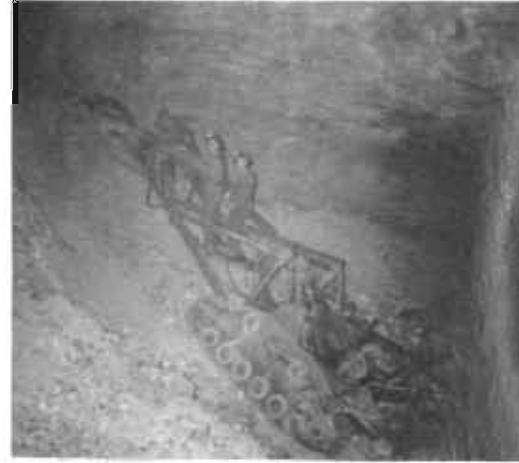
Fig. 3. Drilling in High Ground
