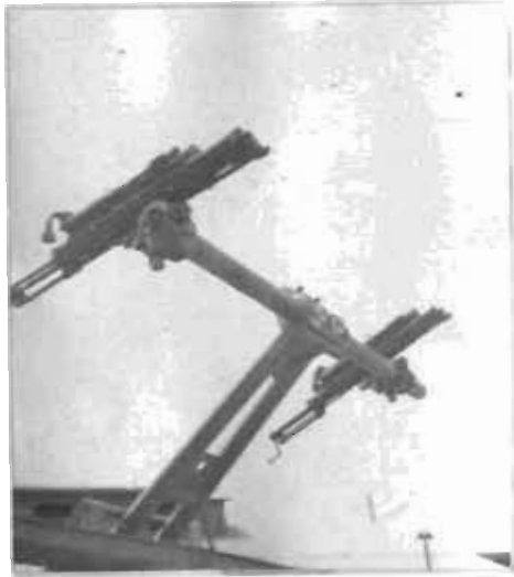
Fig. 1. Drills, Arm, Boom, and Footstand.
