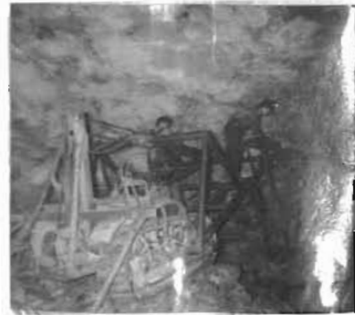
Fig. 4. Setting Up, Breast Hole.
